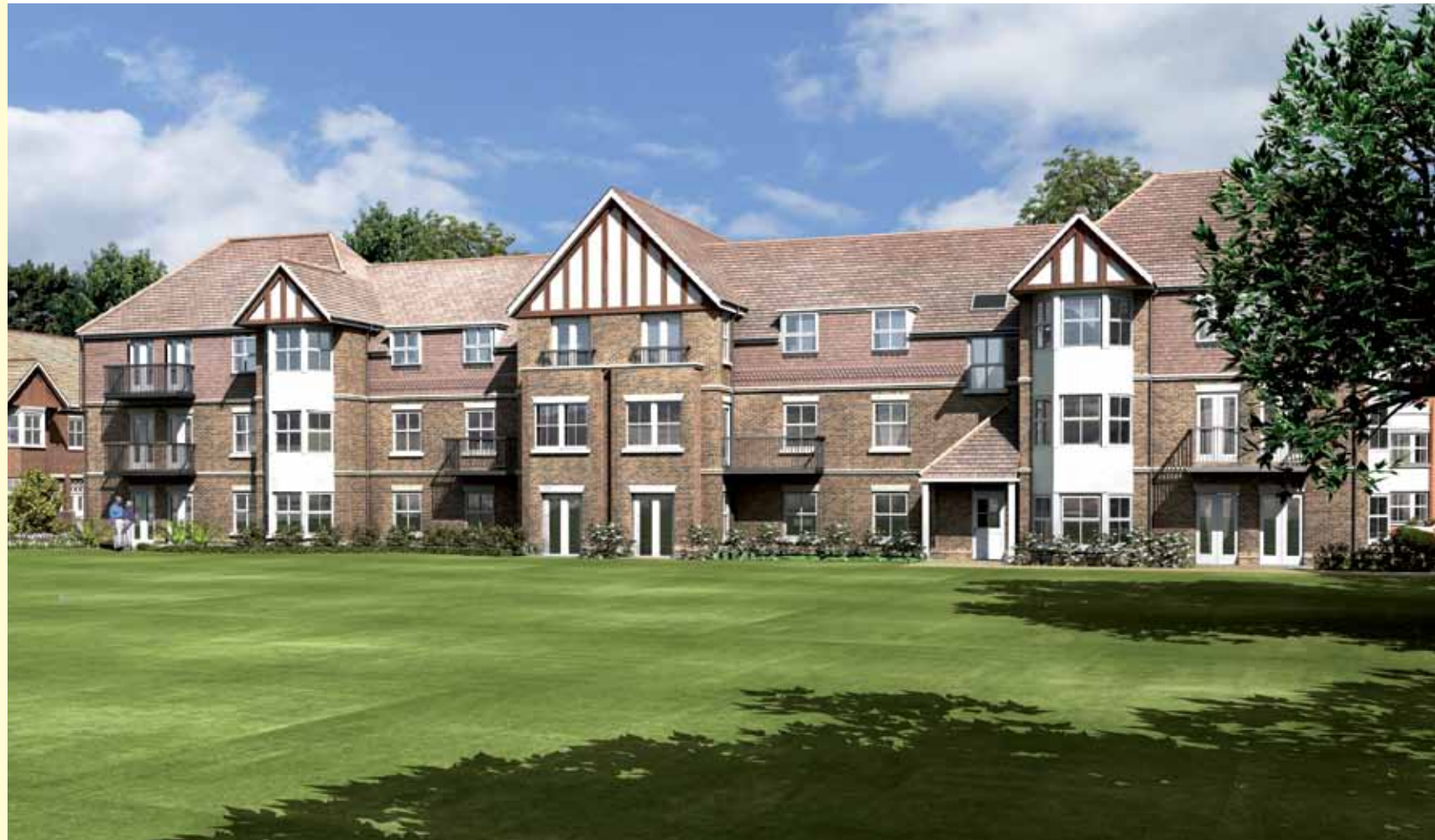
Image shows typical view of large apartment block.
